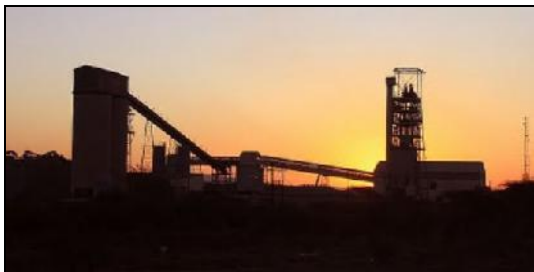
Anglo Platinum – Sunset at Frank Shaft
