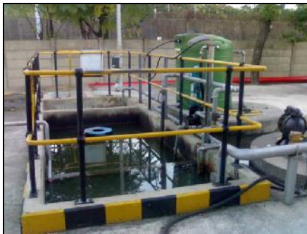
Separator Pits on site
